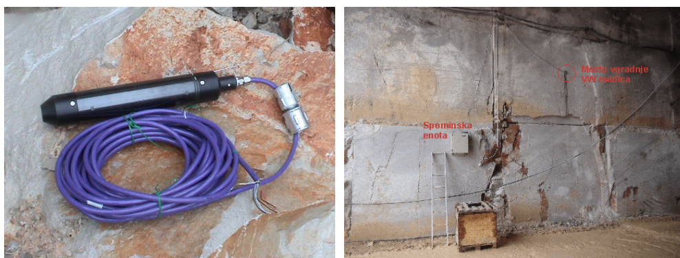
Figure 8.: 2D stress meter (VW biaxial stressmeter 4350BX) (left) and location of installation in the borehole \phi 60\text{mm} in the G1 gallery (right).
