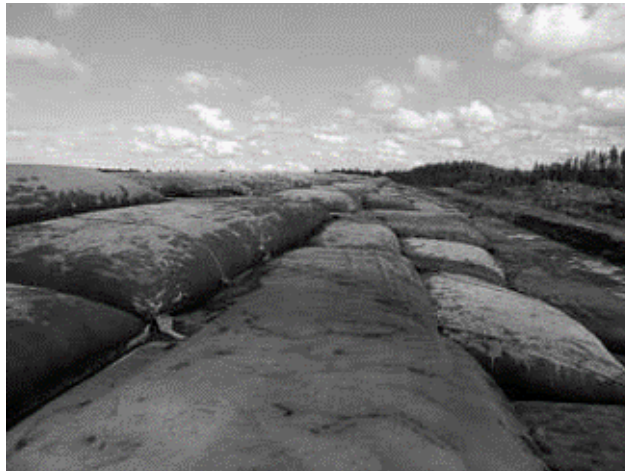
Figure 1 Complete dewatering field showing with fifth tube layer, Wilke & Breytenbach (2015)
